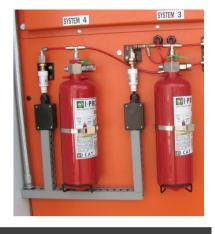
The **I-PROTECT** low pressure automatic fire suppression system consists of a cylinder. detection tube and accessories kit.
