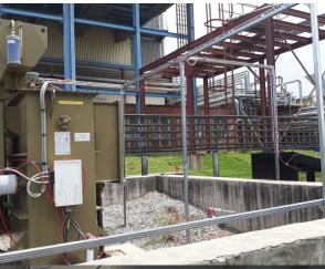
Foam mist as a suppression agent is effective in displacing oxygen through its rapid expansion by coming into contact with the radiated heat from a fire, forming an inert environment. Through its gradual cooling properties, it controls the risk of re-ignition and the spread of a potentially devastating fire. The foam mist prevents thermal shock and poses no threat to hot surface equipment that may crack or damage through rapid cooling. The systems have a Class A, B and C classification.
